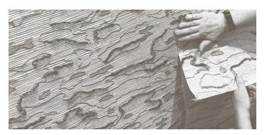
Apply appropriate paste evenly, especially near edges, to the back of the wallcovering, taking care not to get adhesive on face of wallcovering. Allow wallcovering paste to become tacky prior to hanging – timing will vary depending on the temperature and humidity of the room.
