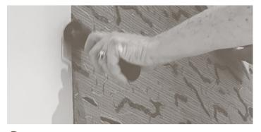
(4) Hang wallcovering with panels side-by-side, noting the "TOP" of each panel. Panels should align – matching pattern.
